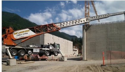
Howard Hanson Dam Seattle, WA
