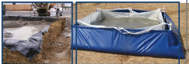
Immovable washout pits
