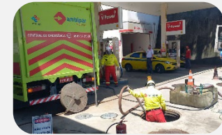
Underground Gas Tank Cleaning
