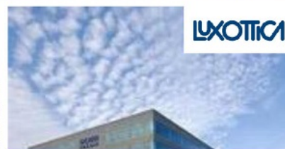
Luxottica Group, US Security and Access Control System
