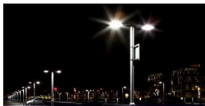
Major Smart Lighting Company, UK Environmental Monitoring
