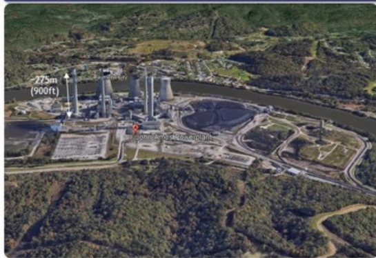
Before: Coal-Fired Power Station
