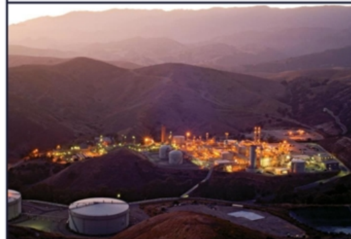
Las Flores Canyon Processing Facility
