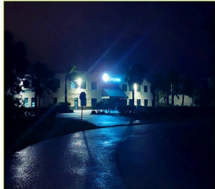
e2 Headquarters during Hurricane Ian powered by R3Di®, Sept. 28, 2022
