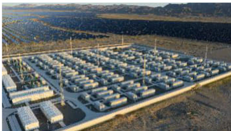
Point Mountain is a multi-technology campus capable of supporting 400 MW of solar and storage, 1,250 MW of natural gas, and a 1000+ MW data center in Crane County, TX
